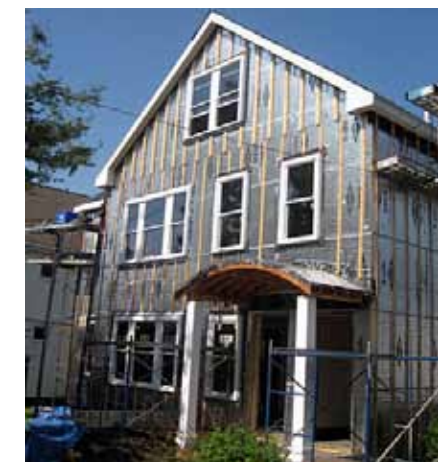
Wrapping the house with foil-faced insulation
